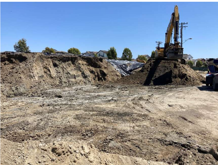
Excavator moving soil to load trucks form stockpile.
