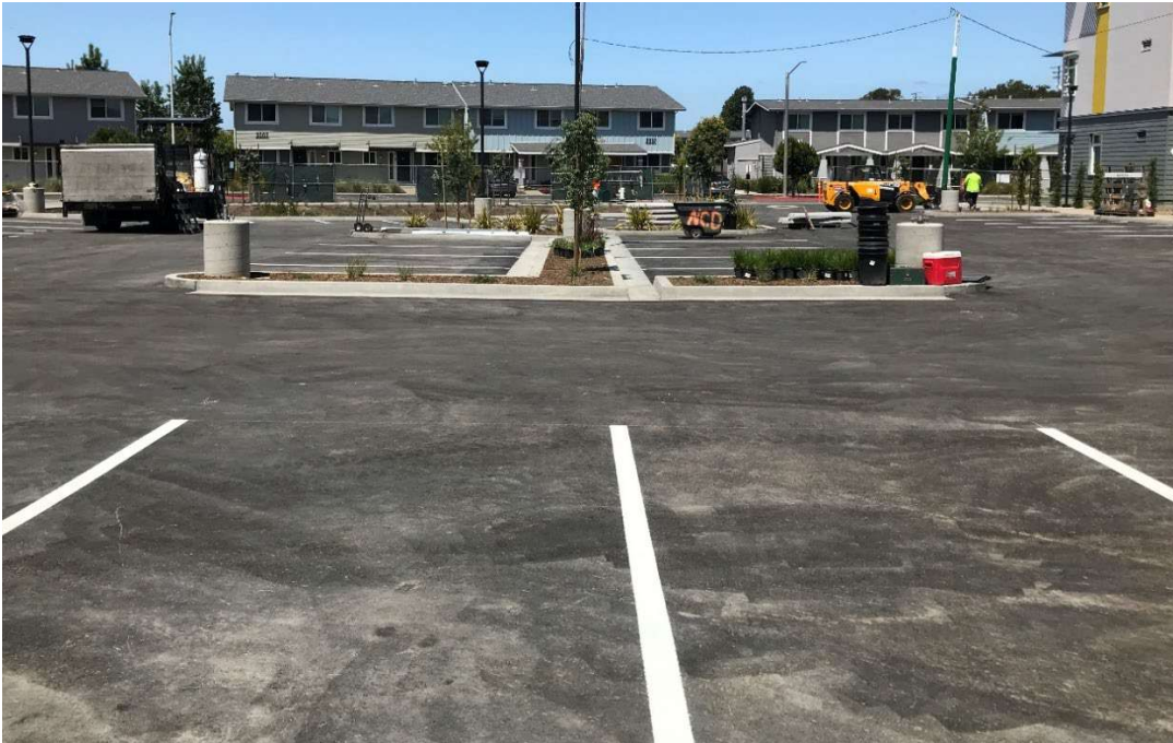
Figure 8: Painting and striping within parking lot areas
