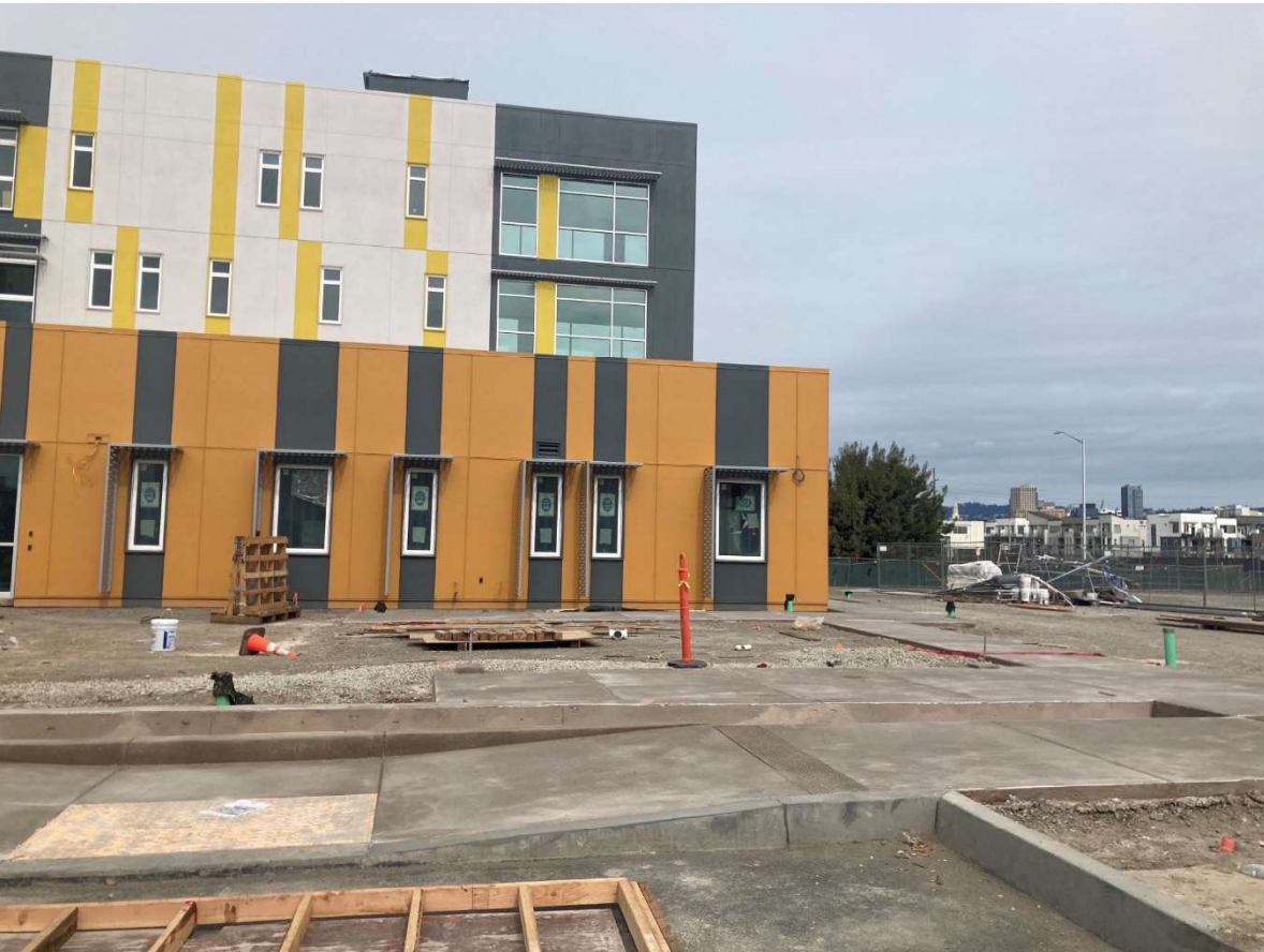
Courtyard cement forms and pours completed.
