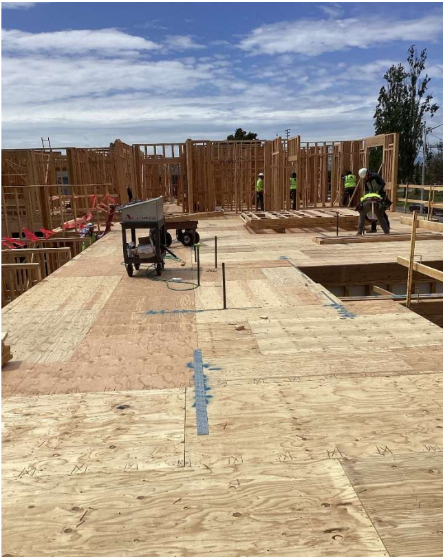
Second floor subfloor installation.
