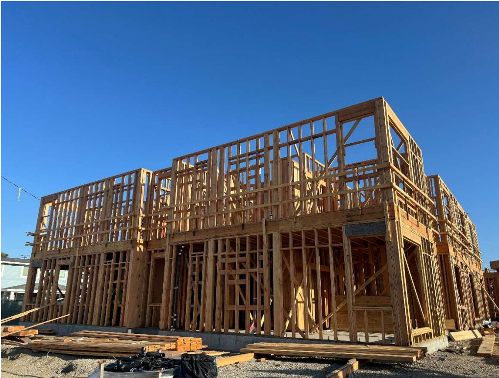
Framing progress photo from the southern elevation.
