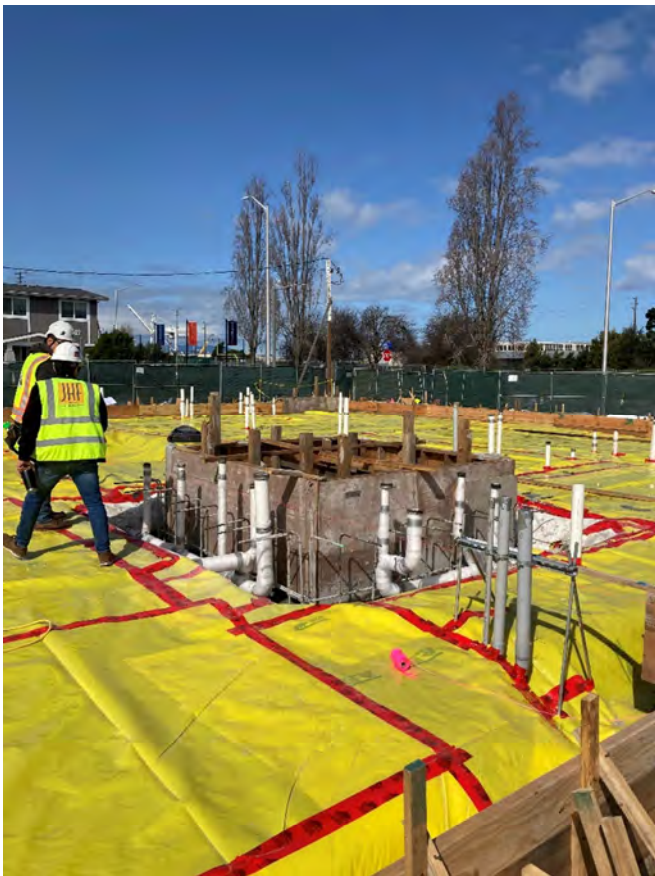
Formation and waterproofing of the elevator pit.
