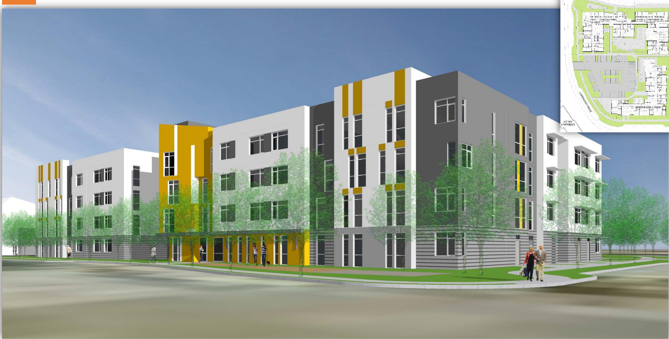
View Looking West from Mosely Avenue
